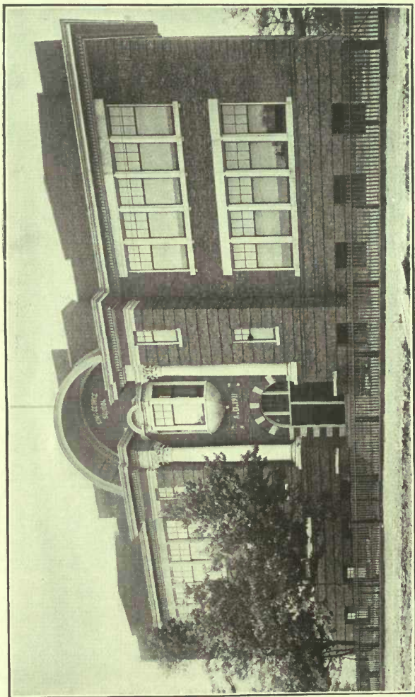
King George School, St. John's Road, for which we manufactured 2 columns, 30 in. in diameter, 22 ft. 6 in. long.
