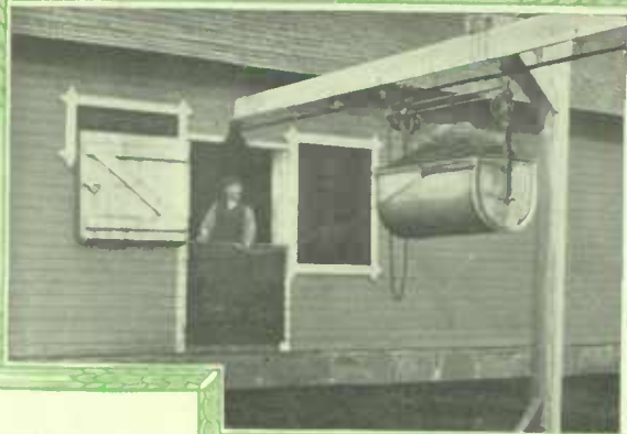
Track arranged with slight incline so carrier may be emptied with trip rope and returned to barn. A barn in Sweden.
