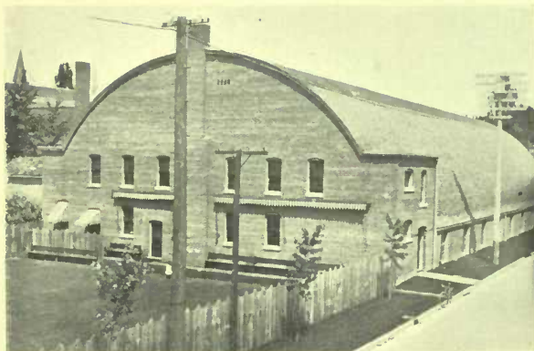
OUTSIDE VIEW OF QUEEN CITY RINK, TORONTO. Showing front elevation.
