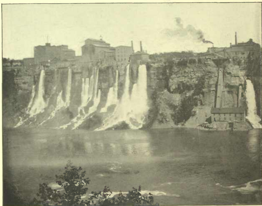
A VIEW OF THE OLD MILLING DISTRICT.
