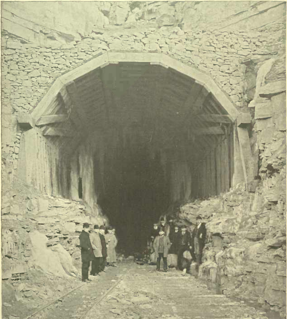
THE MOUTH OF THE TUNNEL DURING CONSTRUCTION.
