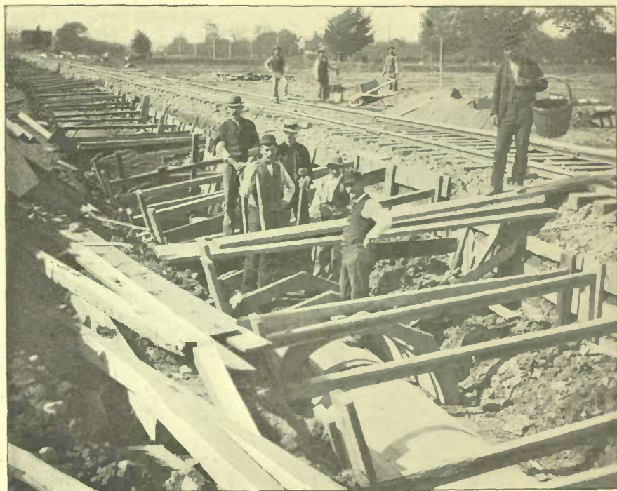
PUTTING DOWN CABLE CONDUITS AT NIAGARA.
