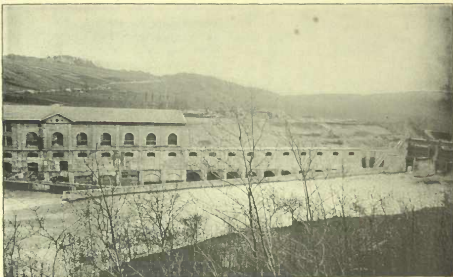
THE NEW POWER HOUSE NEAR GENEVA, CONTAINING 15 TURBINES OF 1200 HORSE-POWER EACH.
