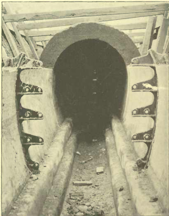
CROSS SECTION OF A CABLE CONDUIT.
