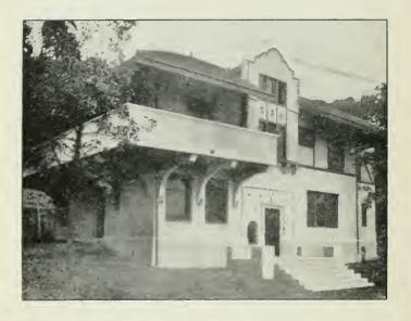
The above is a half-tone of one of many reconstructed residences in Toronto. It was originally an ordinary brick residence, but the bricks having scaled and sheared, expanded metal was attached to them and the whole exterior plastered with cement. The plate speaks for itself.
