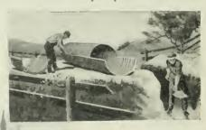
you see the cross-the-road ditch being dug while one man readily clamps the sections together—breaking joints
