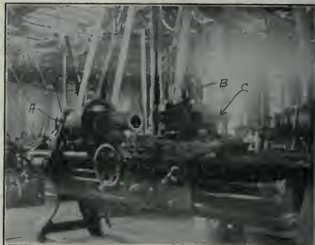
FIG. 4. MACHINING CAST IRON BALL RINGS.
