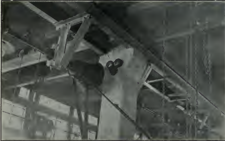
FIG. 2. CRANE BRACKET AND SHAFTING ARRANGEMENT.
