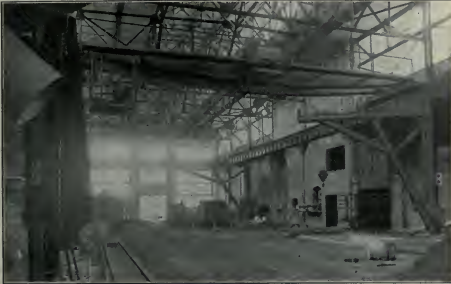
SECTION OF FOUNDRY SHOWING CUPOLAS, CORE AND DRYING OVENS.
