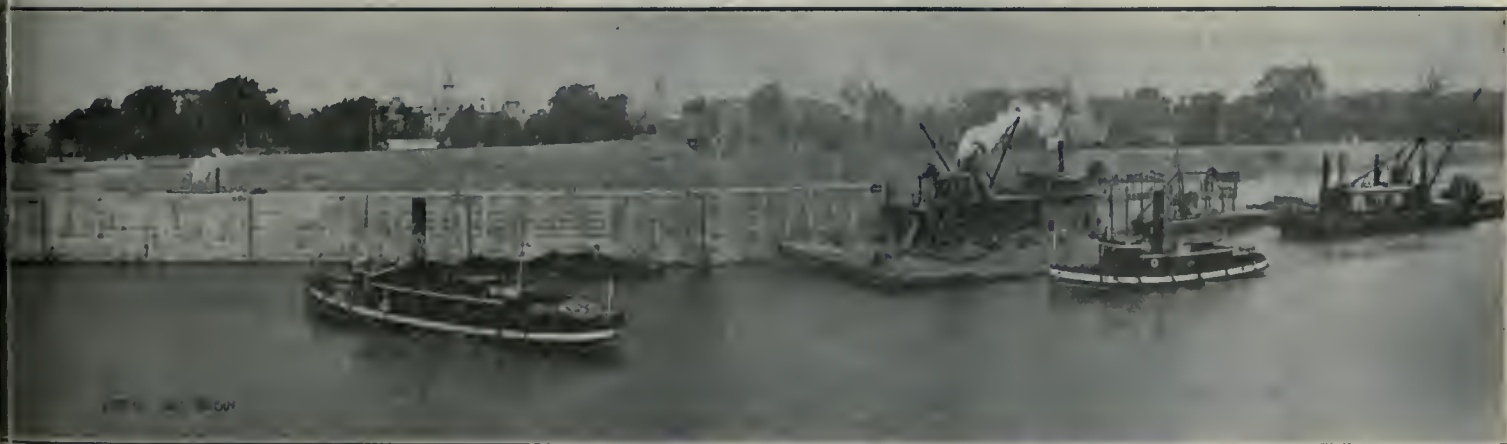
E, MONTREAL. MOST OF THE LAND COMPRISING THE SITE CONSISTS OF MADE GROUND, SOME OF IT BEING SPOIL (ABOUT 2,000 McARTHUR CONCRETE PILES, 16 INCHES IN DIAMETER BY 30 FEET LONG. THE SHIPBUILDING SLIPS WILL TRACTOR, THE PILING CONTRACT HAVING BEEN SUB-LET TO THE McARTHUR CONCRETE PILING CO., NEW YORK.
