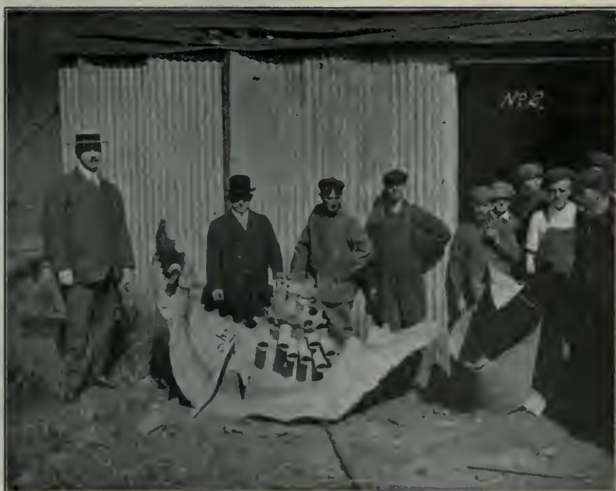
FIG. 2. REAR HEAD AND DOME OF EXPLODED BOILER.
