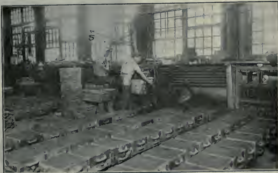
FIG. 15. SPLIT PATTERN SQUEEZERS AND "SUCKER" MOLDING MACHINES (5). BLAKE & KNOWLES FOUNDRY.
