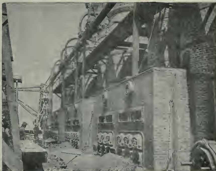
BOILER BATTERY PREVIOUS TO ERECTION OF BOILER HOUSE.
