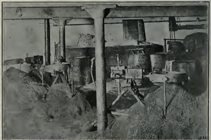
FIG. 11. PREPARING CORE SAND WITH PNEUMATIC RIDDLES.
