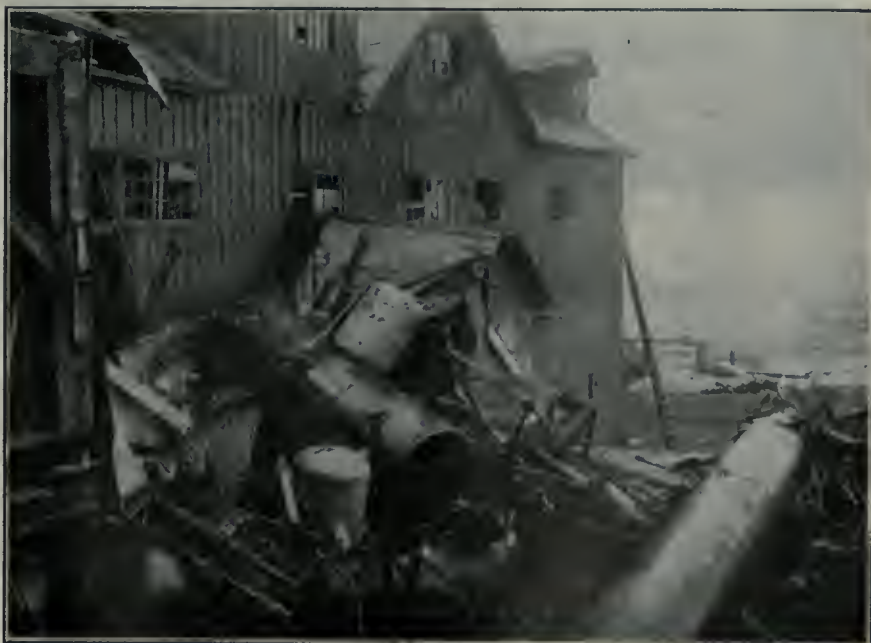
FIG. 4. SHOWING NO. 3 BOILER ON TOP OF NO. 4.
