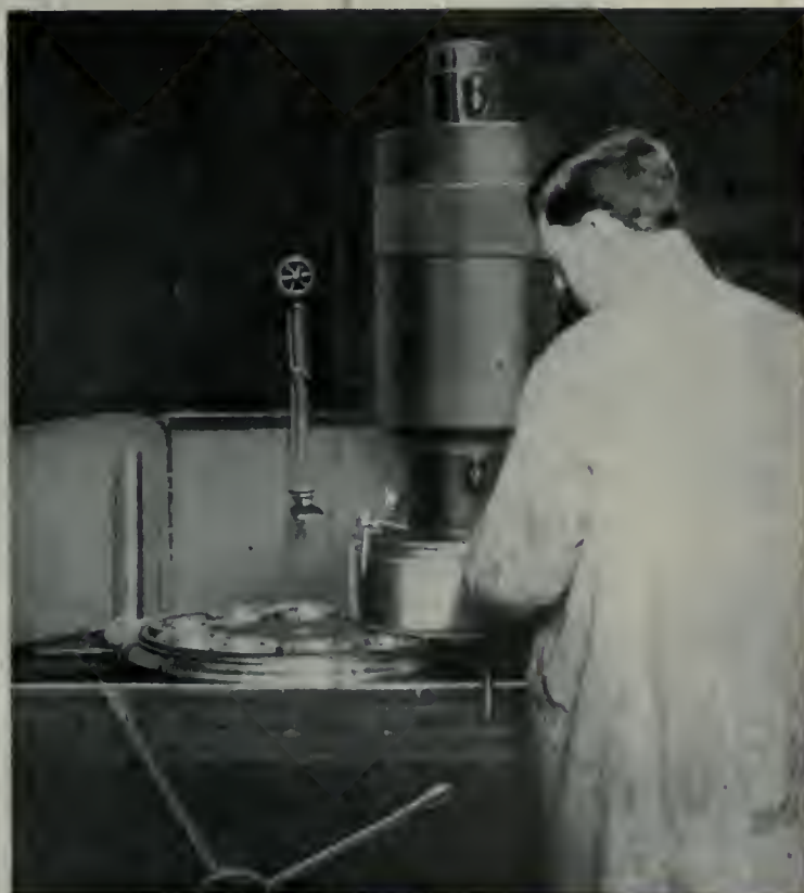
FACING BRONZE BALL CAGES ON A BLANCHARD HIGH-POWER SURFACER.
