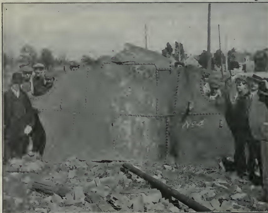
FIG. 4. INSIDE OF PLATES OVER FIRE ON EXPLODED BOILER.
