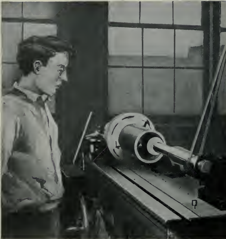
GRINDING A CASE HARDENED SLEEVE ON A LANDIS UNIVERSAL GRINDER.
