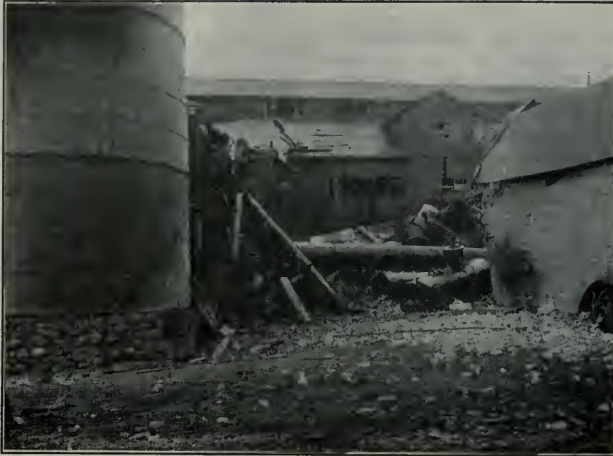
FIG. 1. FUEL HOUSE ON RIGHT, WHICH WAS MOVED SIX FEET. ALSO NO. 1 BOILER AND STACK.
