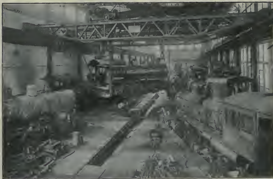
TWO 60-TON OVERHEAD ELECTRIC TRAVELLERS LIFTING A 120-TON LOCOMOTIVE, I.C.R. SHOPS, MONCTON, N.B.
