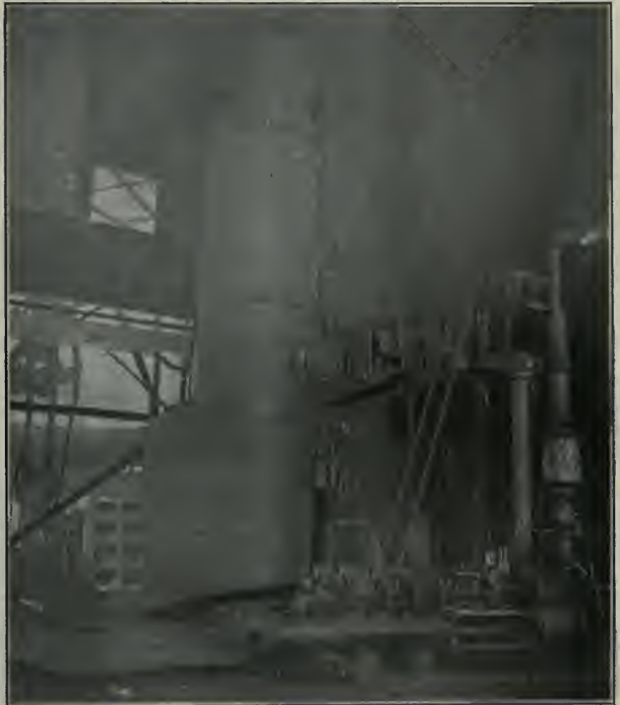
LOCOMOTIVE BOILER SUSPENDED OVER HYDRAULIC RIVETER.
