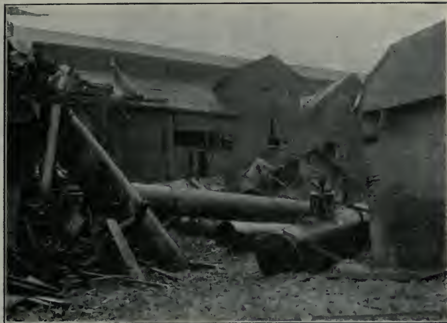
FIG. 3. STEAM HEADER SHOWING THROUGH ROOF OF MILL.
