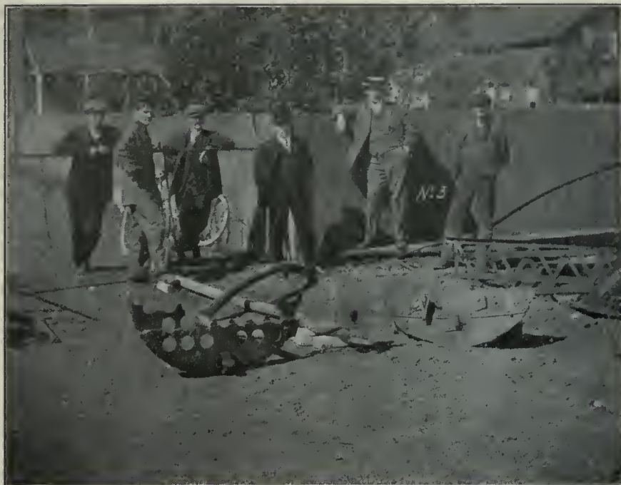
FIG. 3. FRONT HEAD OF EXPLODED BOILER.
