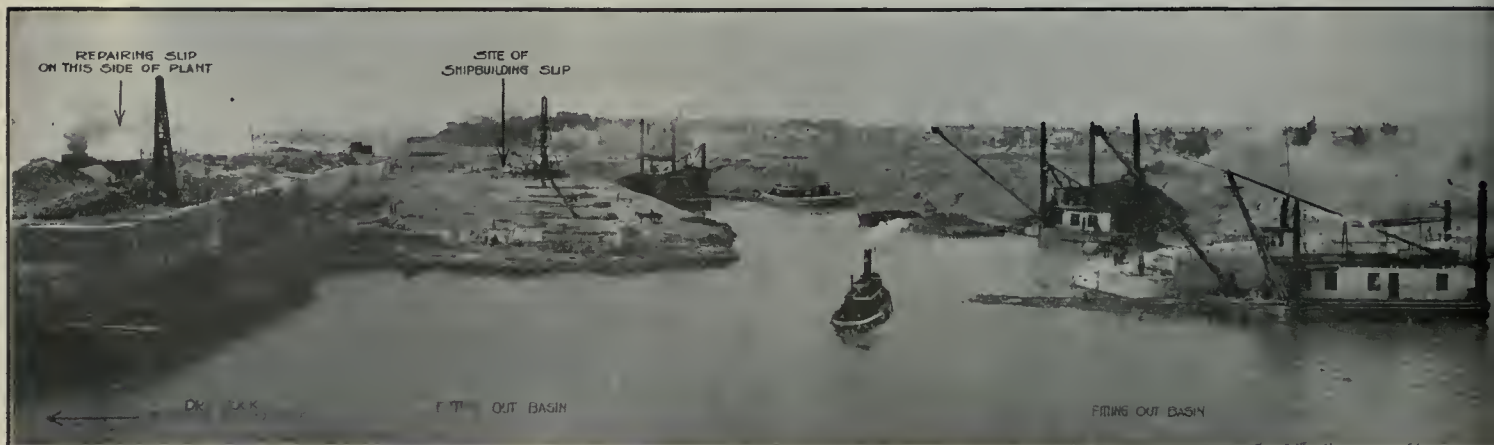
PANORAMIC VIEW OF THE SHIPBUILDING SLIPS AND FITTING-OUT BASIN OF THE CANADIAN VICKERS CO., LTD., AT MONTREAL. THE BASIN WAS DREDGED OUT FROM THE BASIN. WHERE THE VARIOUS BUILDINGS ARE TO BE ERECTED, THE GROUND IS BEING PAVED. IT WILL BE ENTIRELY UNDER COVER, THUS ENABLING WORK TO BE CARRIED ON IN ALL WEATHERS. E. G. M. CAPE IS THE GENERAL MANAGER.
