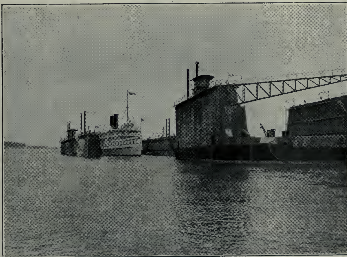
FIG. 1. R. & O. RIVER STEAMSHIP "MONTREAL" ENTERING TWO SECTIONS OF THE FLOATING DRYDOCK.
