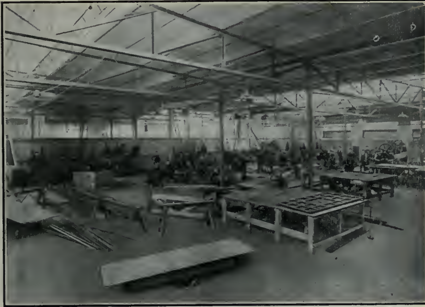
STEEL SASH SHOP.
