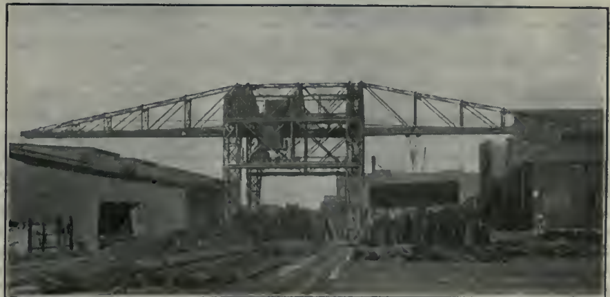
DOUBLE CANTILEVER ELECTRIC TRAVELLING GANTRY CRANE.
