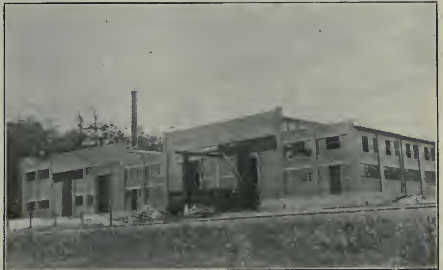
CANADIAN BUFFALO FORGE PLANT EXTERIOR, LOOKING SOUTH.
