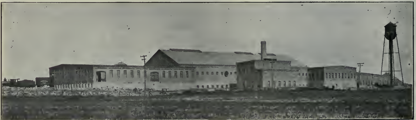
ONTARIO PAPER CO. PLANT, THOROLD, ONT.
