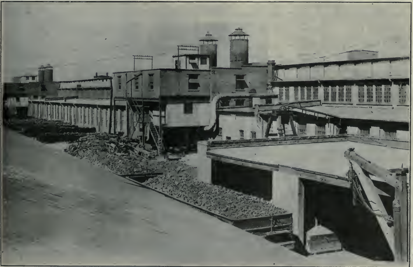
GENERAL VIEW OF PLANT FROM SOUTH SIDE SHOWING STOCK PILES.
