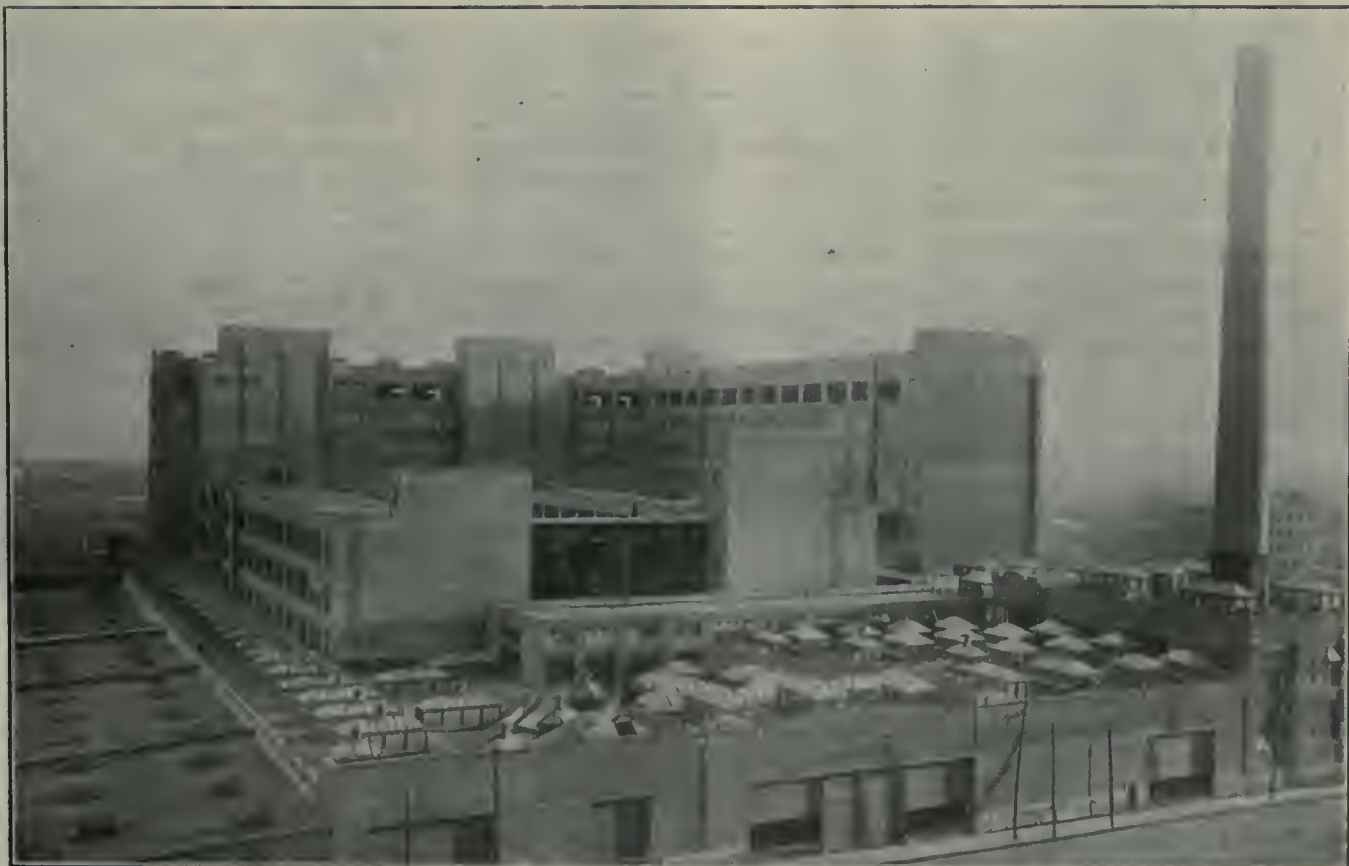
NEW WIRE AND CABLE PLANT, NORTHERN ELECTRIC CO., MONTREAL.
