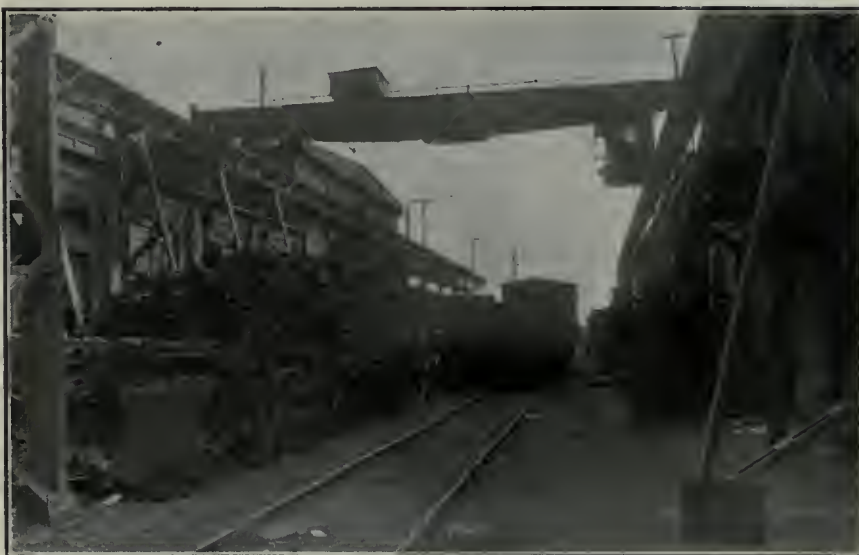
EXTERIOR OF GREY IRON FOUNDRY SHOWING SCRAP PILE.
