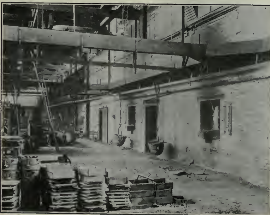
TAP HOLES SHOWING ALSO MONORAIL SYSTEM WITH POTS.
