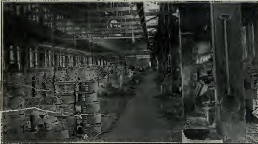
GENERAL VIEW OF EAST WING SHOWING RUNWAY.
