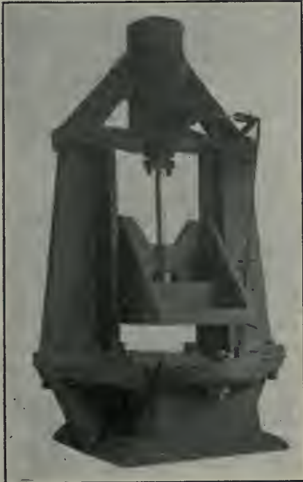
STEAM OR AIR LIFT DROP PRESS.
