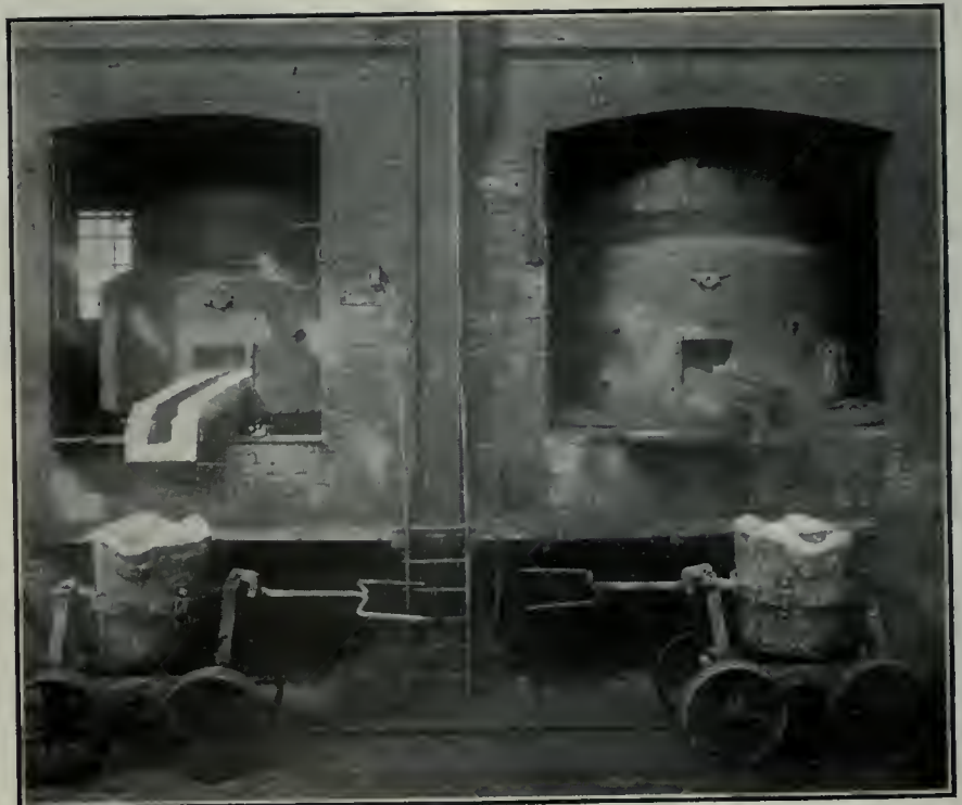
INTERIOR OF GREY IRON FOUNDRY SHOWING CUPOLAS.
