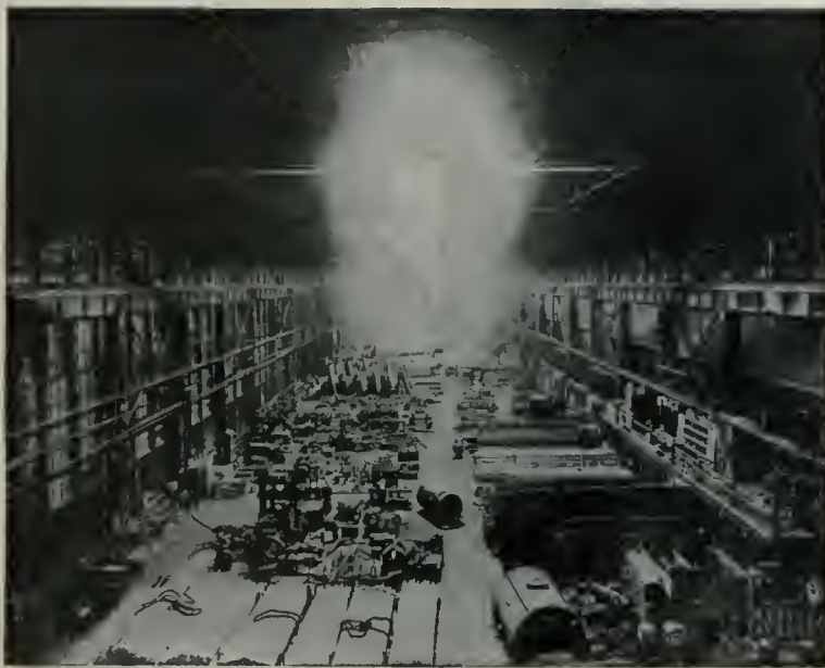
LOCOMOTIVE BOILER SHOP ARTIFICIALLY LIGHTED.
