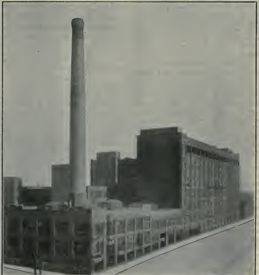
NEW WIRE AND CABLE PLANT, NORTHERN ELECTRIC CO., MONTREAL.
