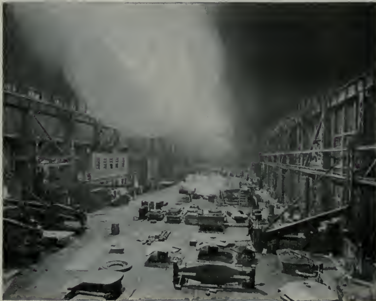
LOCOMOTIVE BOILER SHOP ARTIFICIALLY LIGHTED.
