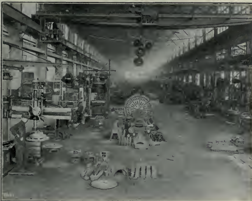
INTERIOR OF PORTION OF C.P.R. "OGDEN" SHOPS, CALGARY, ALTA.
