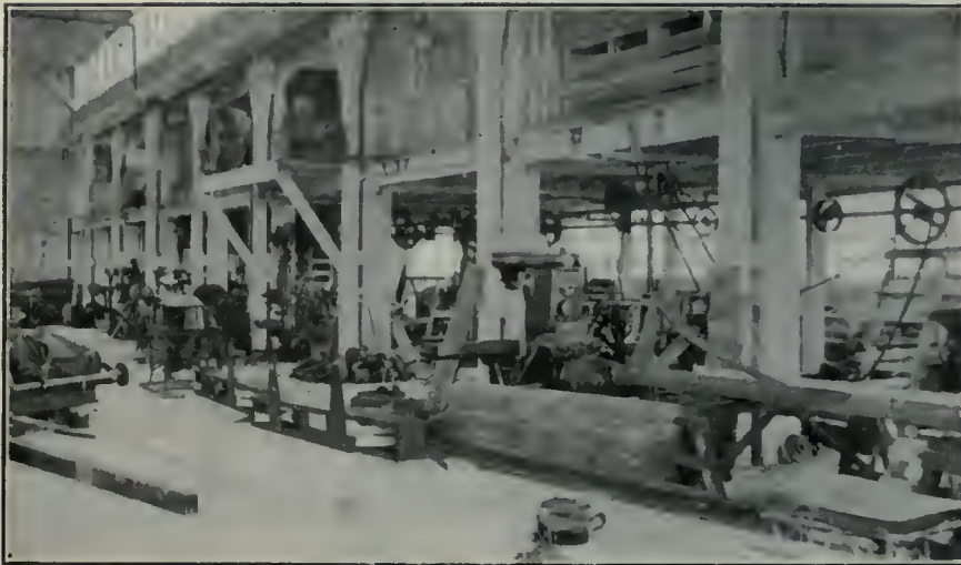
ERECTING BAY, GALLERY AND MACHINE SHOP, LOOKING SOUTH.
