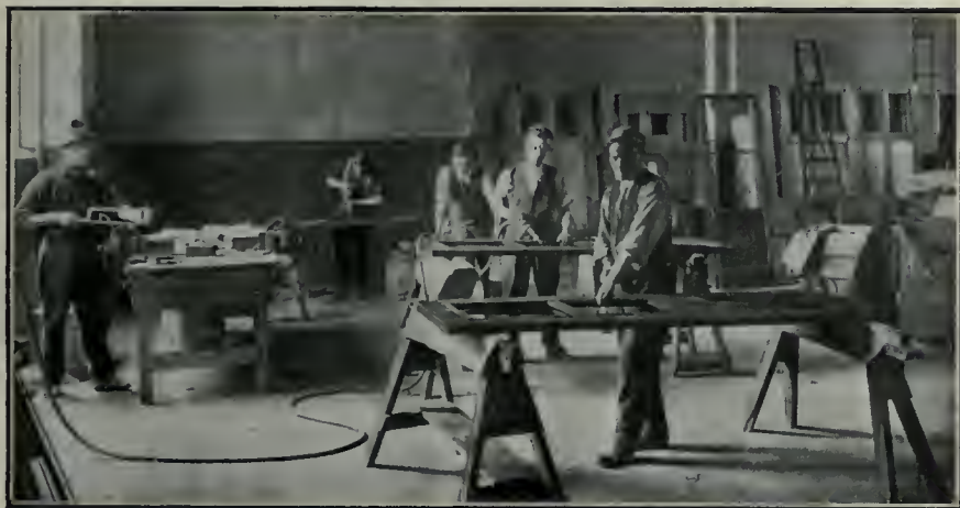
ASSEMBLING HOLLOW STEEL DOORS.
