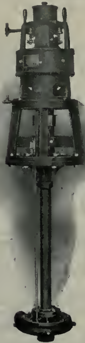
VERTICAL CENTRIFUGAL PUMP.
