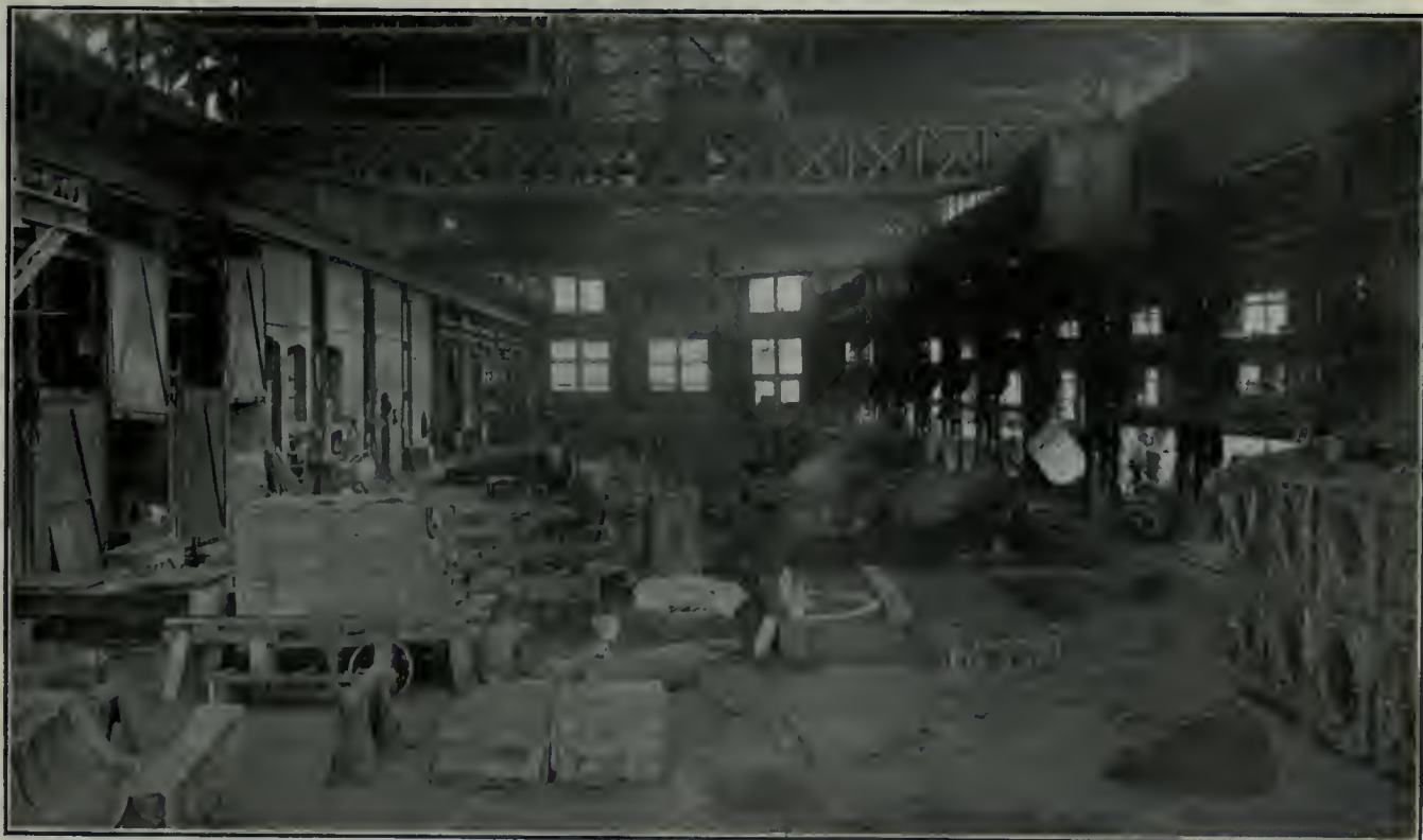
GENERAL VIEW OF INTERIOR OF GREY IRON FOUNDRY.
