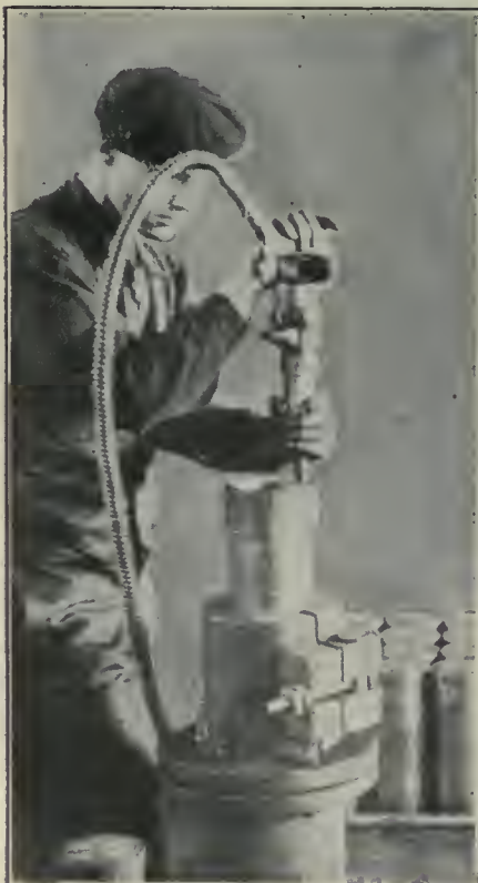
FIG. 12. RIVETING-IN BASE PLATES.
