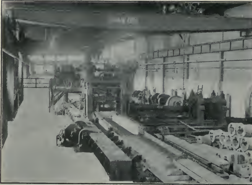
ELECTRICALLY-DRIVEN REVERSING BLOOMING MILL.
