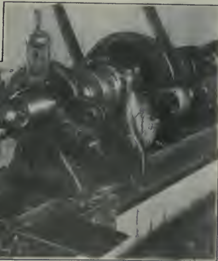
FINISHING BRASS SOCKET AND FORMING FUSE SEAT.
