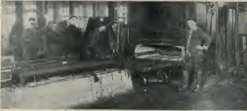
FIG. 4. ANNEALING FURNACES SHOWING CHARGING ARRANGEMENT.
