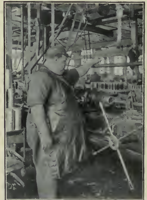
FIG. 10. BORING ON A "JONES & LAMSON" TURRET LATHE.
