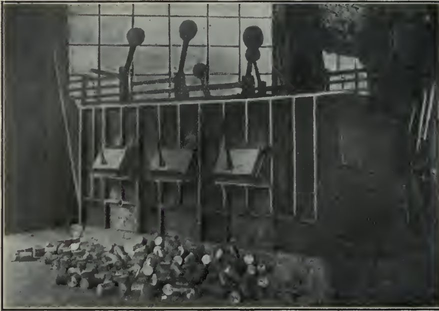
FIG. 3. OIL FURNACE FOR HEATING BILLETS PREVIOUS TO PIERCING OR FIRST OPERATION.
