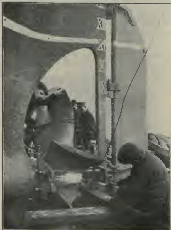
HEATING WITH BLOW-PIPE TO REMOVE PROPELLER
