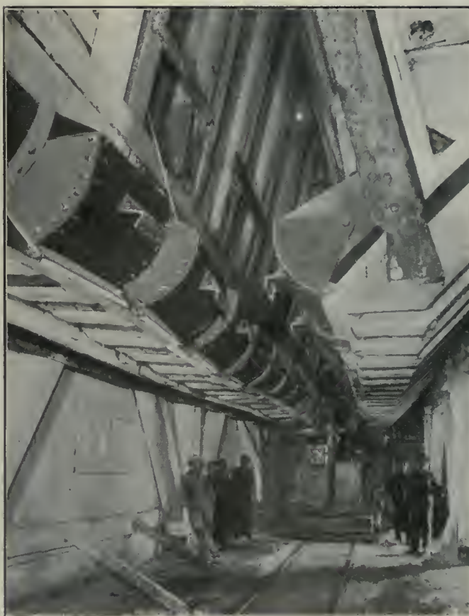
ELECTRICALLY DRIVEN CHARGING CAR WHICH WEIGHS THE ORE, COKE, ETC., AS DELIVERED BY OVER-HEAD CHUTES FROM CHARGING BINS.
