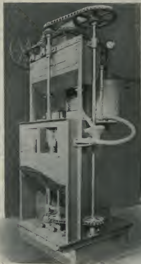
SHRAPNEL SAND BLASTING MACHINE.
