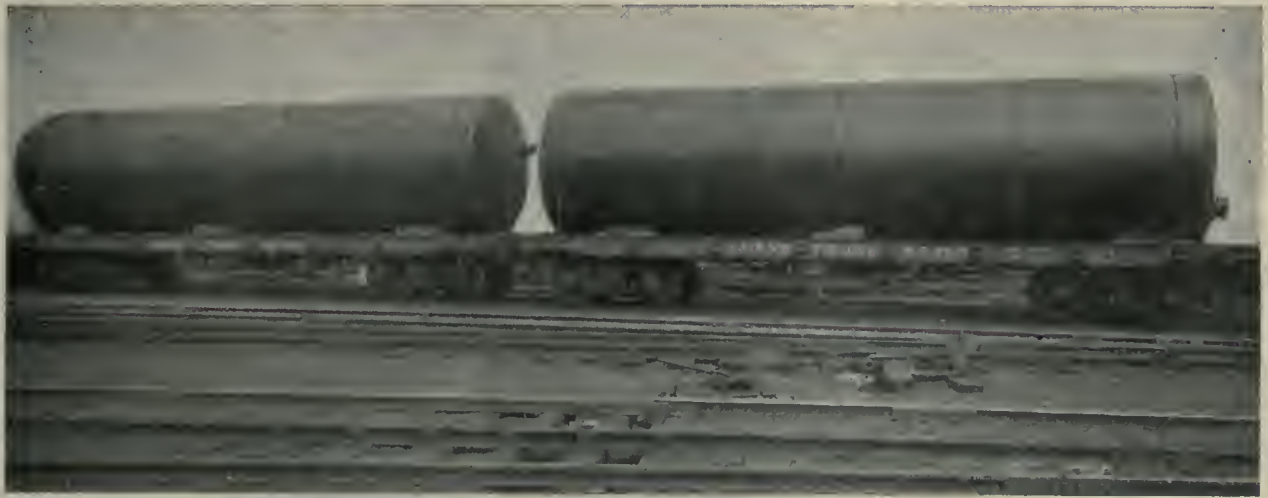
Pressure Filter Tanks for one of the Western Municipalities
