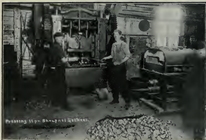
FORGING BRASS SOCKETS FOR SHRAPNEL IN A POWER PRESS.
