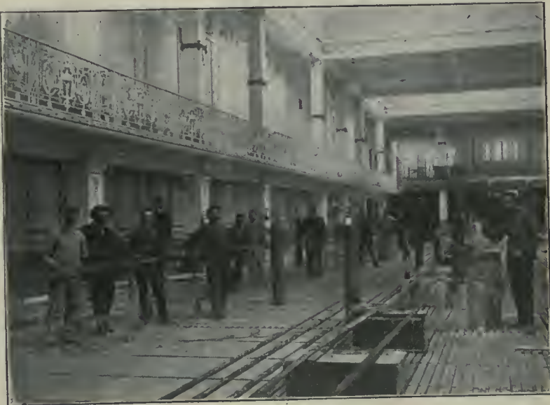
INSTALLING FREEZING COILS WITH WELDED JOINTS IN AN ARTIFICIAL ICE SKATING RINK.
