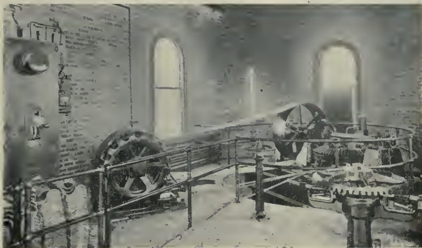
FIG. C. LOW LIFT McDUGALL SUBMERGED CENTRIFUGAL PUMP, BELT-DRIVEN FROM A 75 H.P. WESTINGHOUSE INDUCTION MOTOR.
