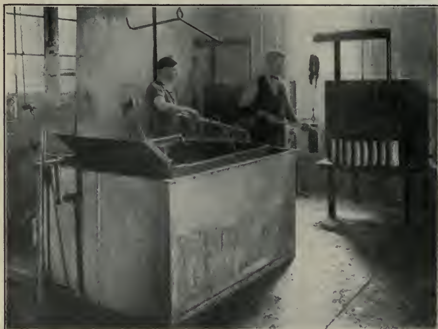
FIG. 4—HARDENING AND TEMPERING; DOMINION BRIDGE CO. FURNACES
