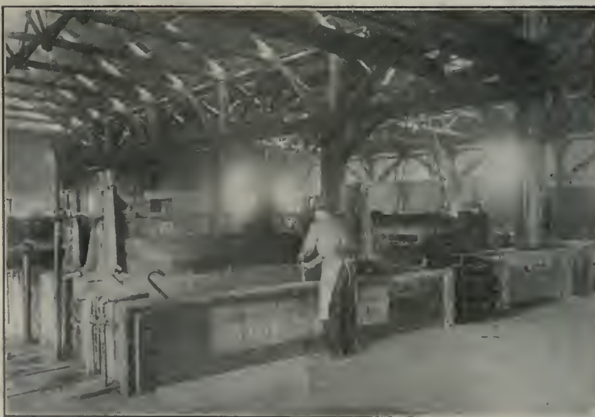
PICKLING DEPARTMENT WHERE SHEETS ARE PREPARED FOR GALVANIZING.
