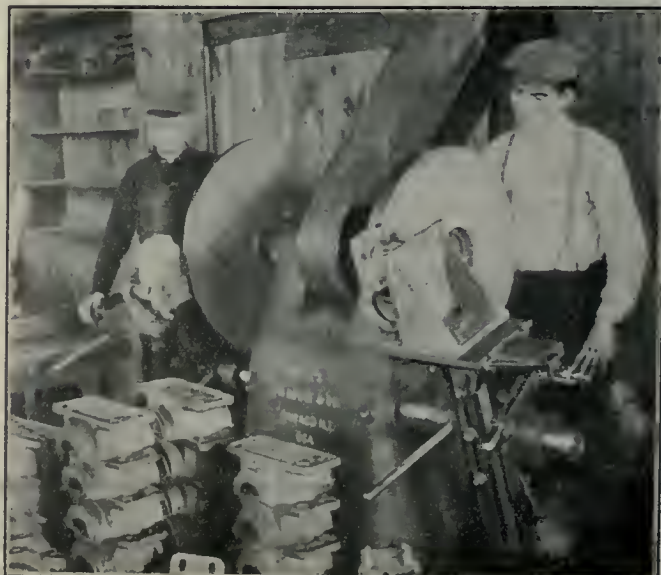
FIG. 2. GRINDING CAST IRON PILLOW BLOCKS AND CAPS.
