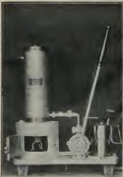
FIG. 2. THE "REICHENBACH" HEATER AND FUEL OIL STARTER.
