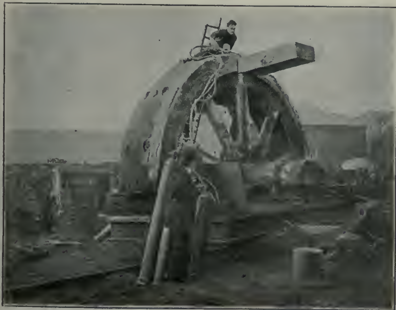
REMOVING RISER WITH BLOW-PIPE.
