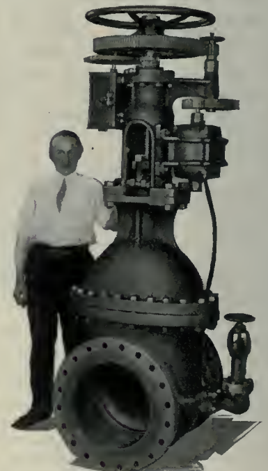
16-IN. MOTOR OPERATED SOLID WEDGE GATE VALVE.
