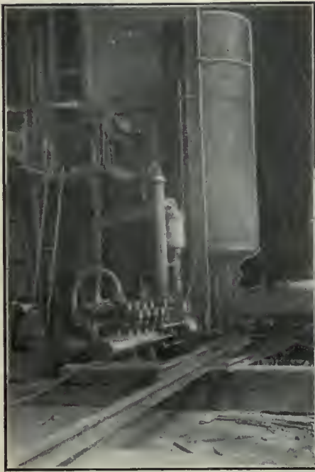
FIG. 13. SNOW STEAM PUMP AND ACCUMULATOR DELIVERING WATER TO HIGH PRESSURE MAINS AT 1,500 LBS. PER SQ. INCH.
