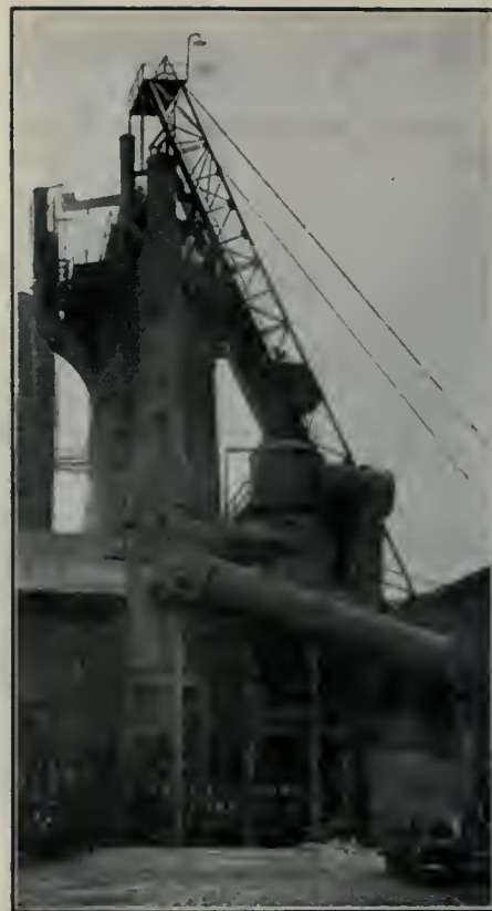
EXTERIOR VIEW OF BLAST FURNACE. SHOWING PIPES FOR CONVEYING WASTE GASES TO STOVES. DUST SEPARATOR IN FOREGROUND.
