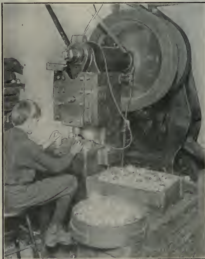
FIG. 8. PRESSING COVER ON POWDER CUP.
