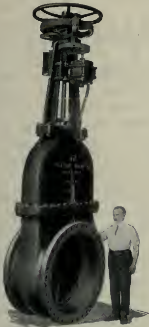
42-IN. MOTOR OPERATED SOLID WEDGE GATE VALVE.
