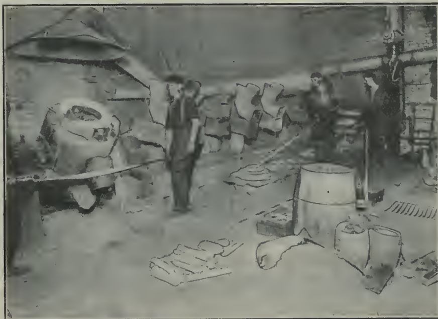
FIG. 1. CRUCIBLE SECTION OF BRASS FOUNDRY WHERE SLUGS FOR FUSE SOCKETS ARE PRODUCED.
