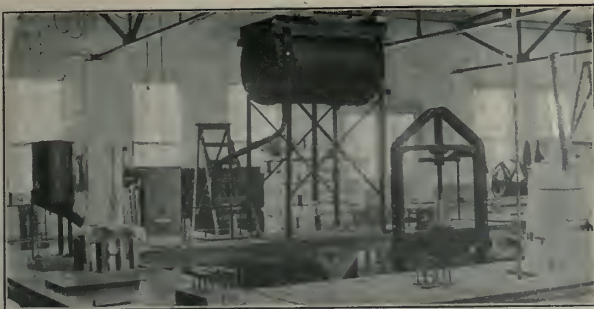
FIG. 12 CHARGING DEPARTMENT SHOWING BULLET HOPPER, POWDER TANK, LOADING PRESS AND RESIN FURNACE
