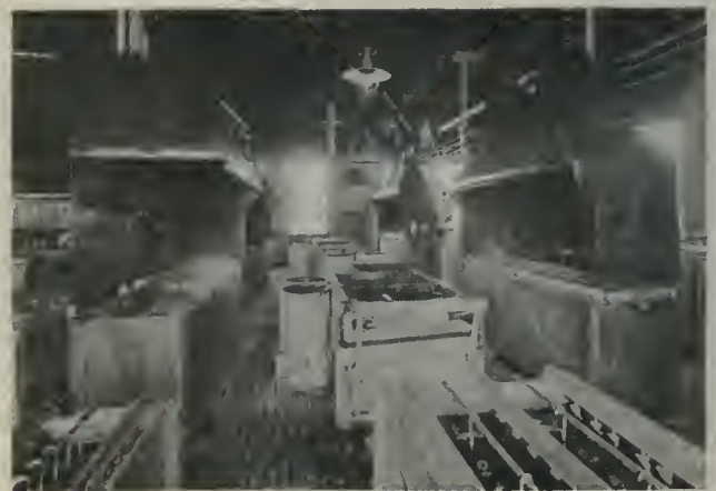
COPPER PLATING AND CLEANING SECTION SHOWING ACID JARS AND SWILLING TANKS.
