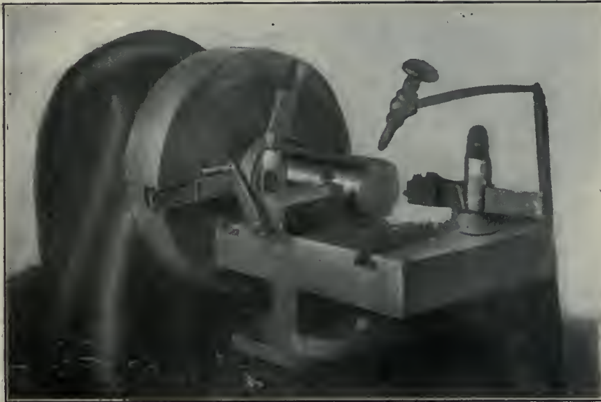
ROUGH TURNING SHRAPNEL SHELL BODIES.
