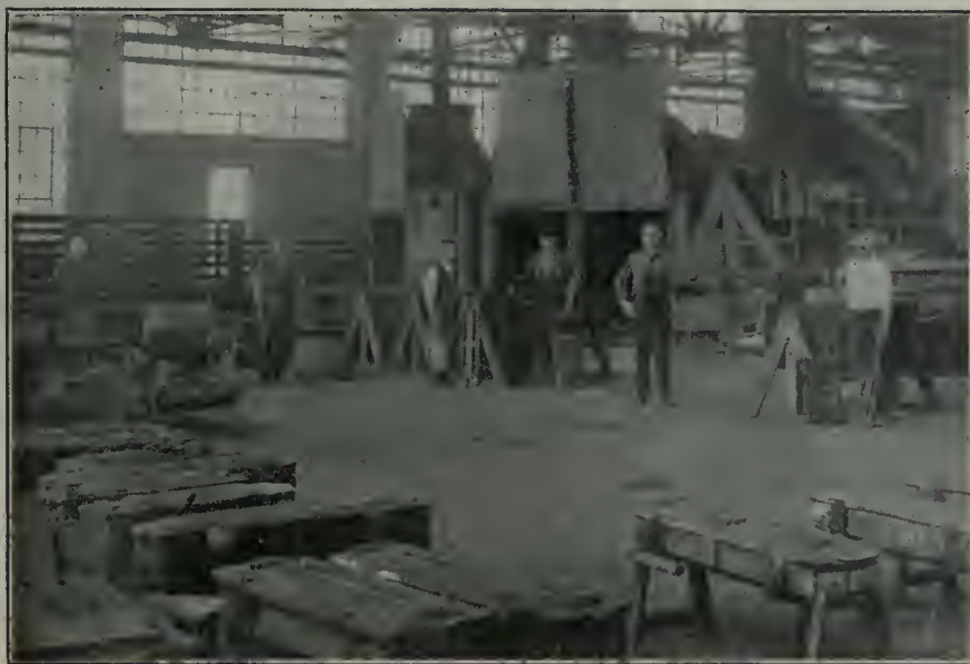
FIG. 1. FINISHED CORE AND CORE OVEN DEPARTMENT.
