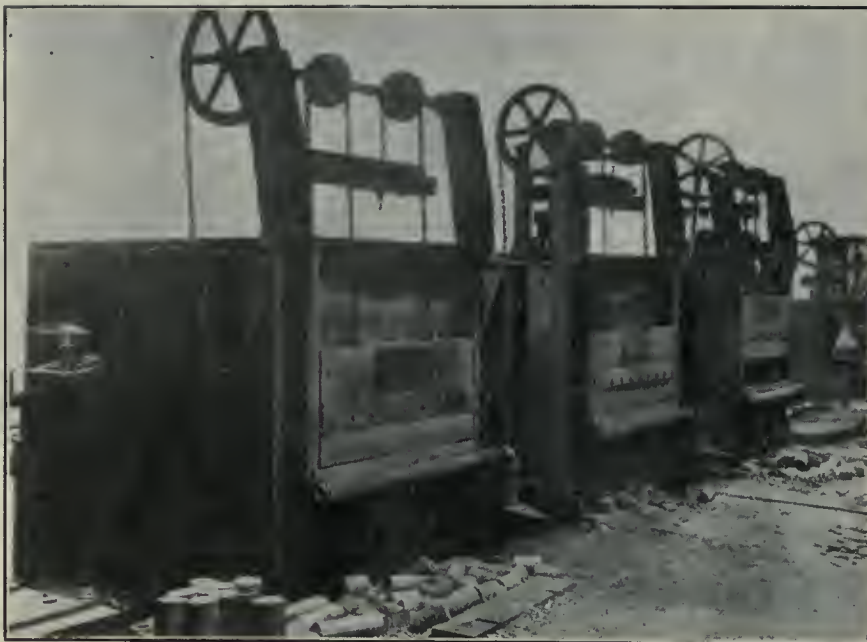
FIG. 2. "MECHANICAL ENGINEERING CO." FURNACES FOR HEATING AND REHEATING BILLETS.
