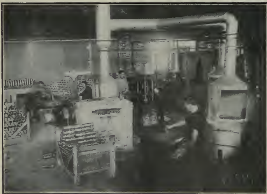
HEAT TREATING DEPARTMENT SHOWING FURNACES, ALSO BANDING AND NOSING PRESSES IN BACKGROUND.
