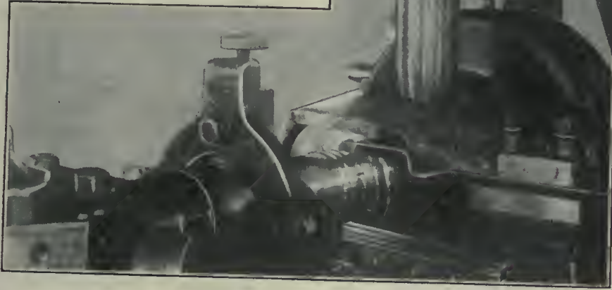
COPPER BAND TURNING.
