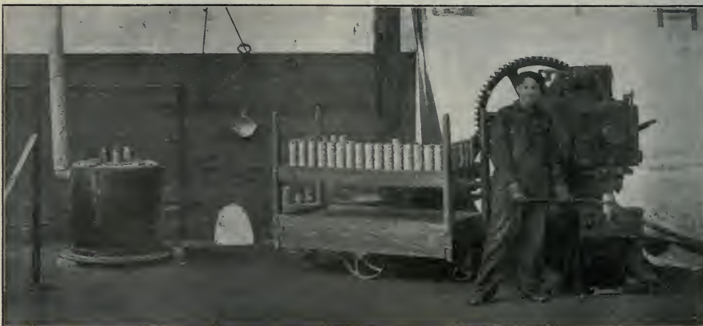
OIL-FIRED LEAD BATH FURNACE AND POWER PRESS FOR FORMING NOSE ON SHRAPNEL.
