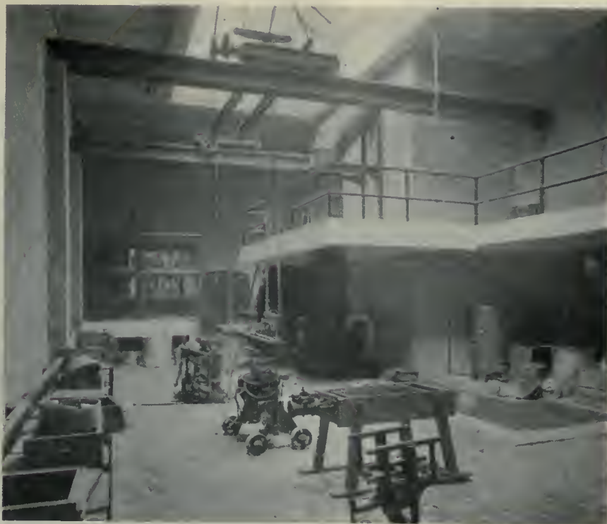
DEPARTMENT OF SHOPWORK. VIEW OF FOUNDRY SHOWING CHAPOLA, BRASS FURNACES, MOULDING MACHINES, AND WORK BENCH.
