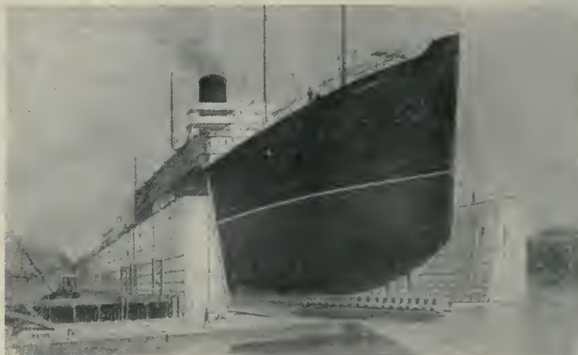
THE NEW FLOATING DRYDOCK WITH A LARGE VESSEL ABOARD.
