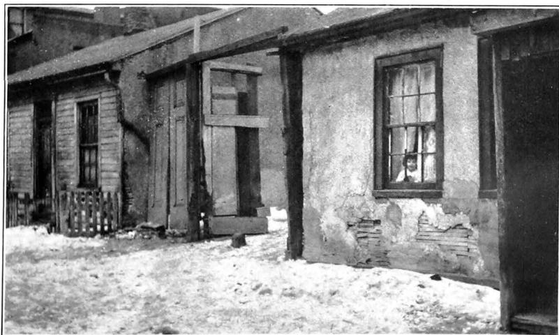
plaster has fallen off, and there is, more or less, an absence of paint or whitewash. Fences about the houses have partly collapsed and no effort is made to repair them or to remove them altogether. Sidewalks leading to the houses and doorsteps are in a broken condition, and the doors themselves are usually in a state of ill-repair. Wooden shutters sag from one hinge or have many slats missing.
