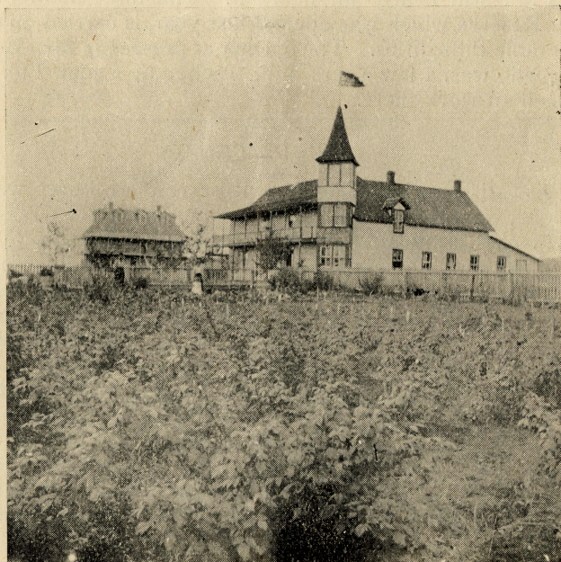
BOARDING SCHOOL, ONION LAKE. TWO MAIN BUILDINGS. ST. BARNABAS' MISSION.
