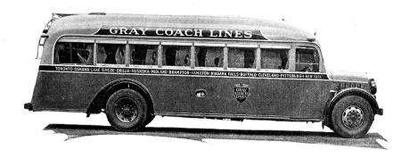
Sleek and silent, these coaches purr along the highways, providing what doe indeed seem to be the last word in safe and comfortable interurban transportation service. Some of its most important features are reclining seats, hot wate heating, forced air ventilation, four-wheel air brakes, enclosed baggage compart ments, and innumerable other devices for the safety and comfort of passengers
