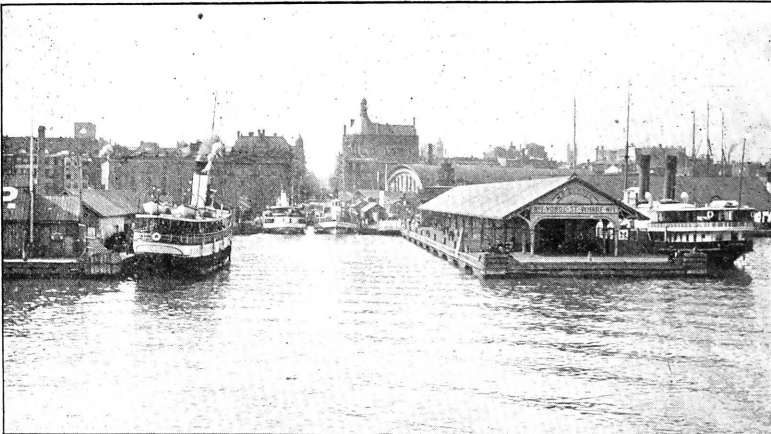
Yonge Street Wharf—from the Bay.
