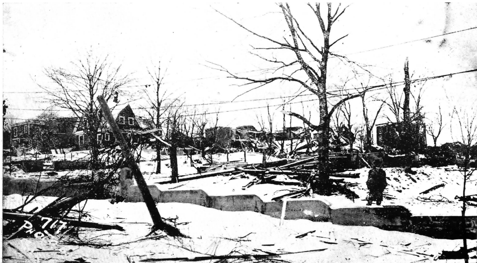
KAYE ST, METHODIST CHURCH WAS BLOWN DOWN AND BURNT. Note foundation in the foreground.
