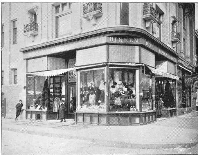
W. & D. Dineen's New Fur Store, Cor. Temperance and Yonge Streets, Toronto Lighted with Luxfer Prisms in Show Window Transoms. F. H. Herbert, Architect.
