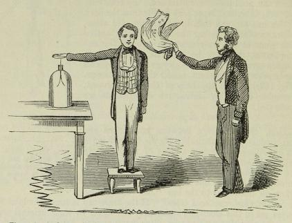
Fig. 170. Assistant standing on the insulating stool and touching the disc of the electroscope whilst being struck with a dry handkerchief.
