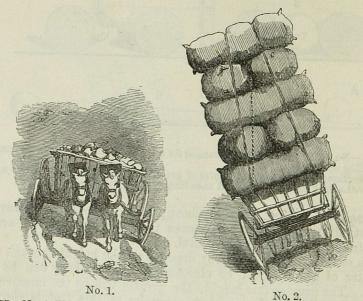
Fig. 57. No. 1. The centre of gravity is near the ground, and falls within the wheels. No. 2. The centre of gravity is much elevated, and the line of direction is outside the wheels. with a very heavy substance which does not occupy much space, such as iron, lead, or copper, or bricks, it will be in much less danger of an overthrow than if it carries an equal weight of a lighter body, such as pockets of hops, or bags of wool or bales of rags.
