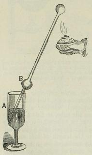
Fig.398 b. Heating and expanding the air in the top bulb, so that when cool the mercury in the glass A, may rise into the tube and fill the bulb B. bag fitted on to the other extremity of the tube. The operator now marks off the intended length of his thermometer, and above that point the tube is again softened with the flame and blowpipe, and a second bulb blown out. (Fig. 398 a.)
