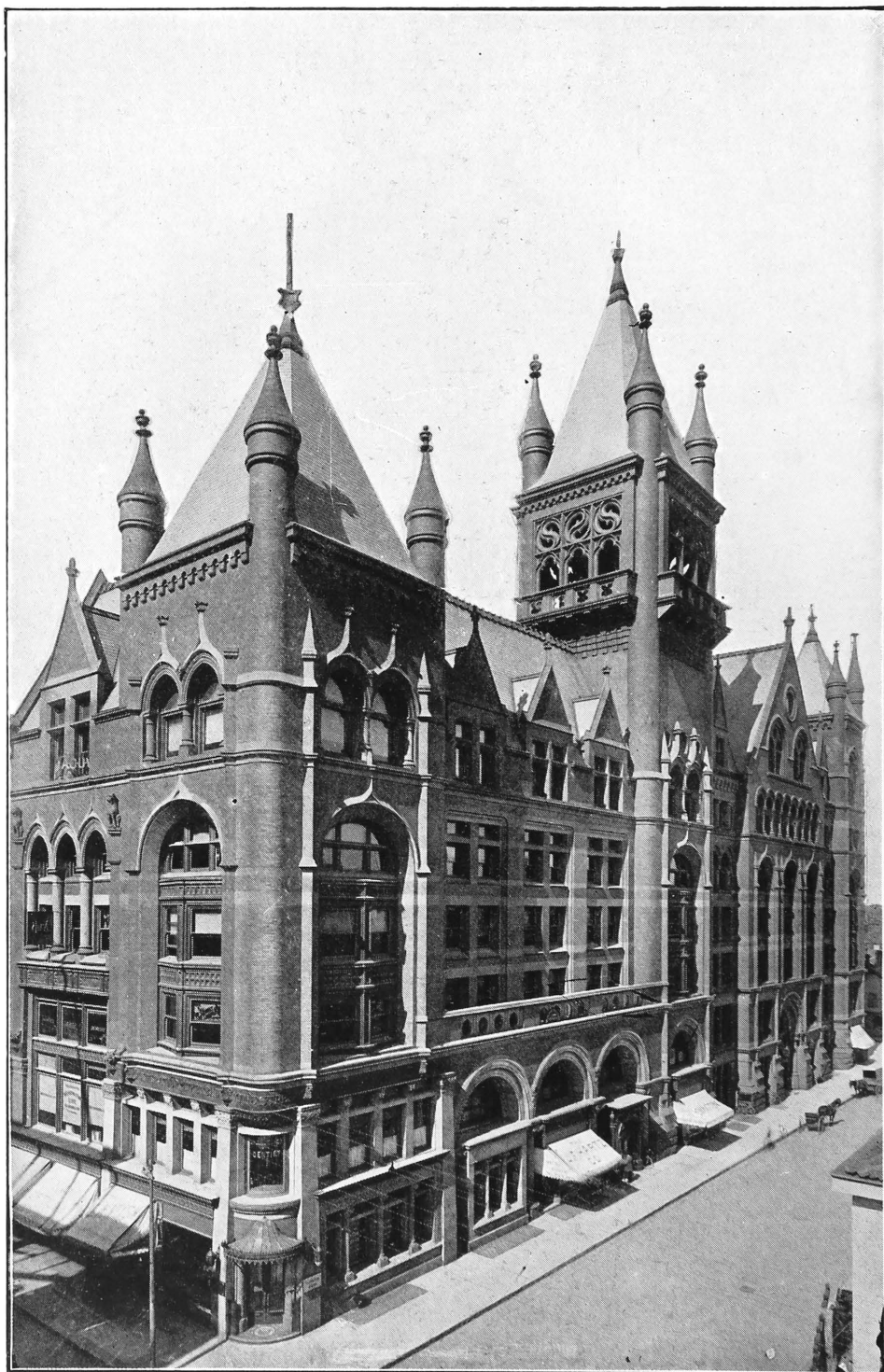
The Confederation Life Building.
