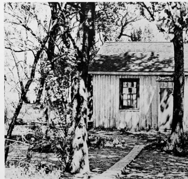
George Lang's Cottage, Cottage 64, Woodbine Beach, 31 May 1916
