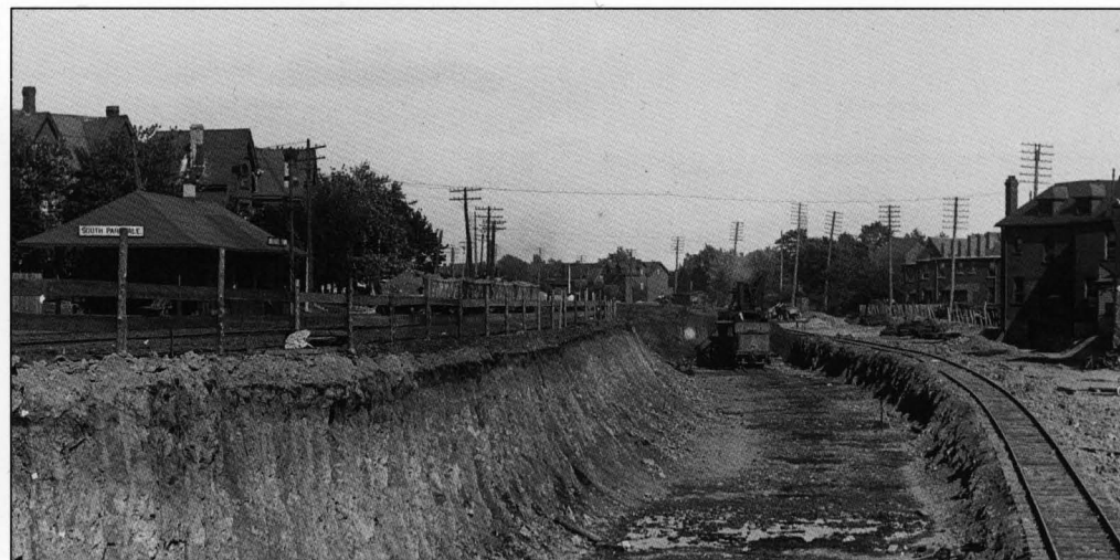
Between 1910 and 1912, the Grand Trunk Railway's line through south Parkdale was placed below grade, in a deep ditch. The work is shown in this 28 June 1911 progress photograph looking east towards Close Avenue. The GRT's South Parkdale Station is on the left. This was one of several projects which contributed to Parkdale being cut off from its Lake Ontario waterfront.
