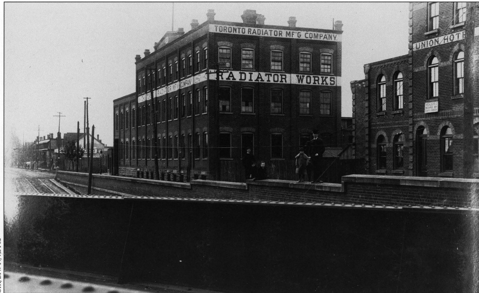
The Toronto Radiator Manufacturing Company is shown in this 7 November 1894 view looking south down Dufferin Street from the subway at Queen. An 1892 publication described its operations: "The premises at Toronto cover some five acres of ground in buildings and yards. The main factory is a splendid four storey brick building, 230 x 510 feet in dimensions. The company have the largest and most complete plant for radiator work to be found on the continent, and they are sole makers in Canada of the Safford patent." 24
