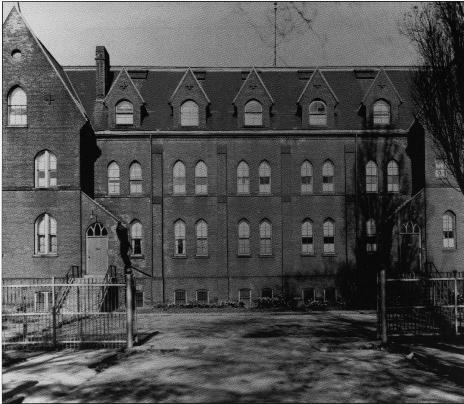
The Sisters of the Good Shepherd built this convent at West Lodge in 1888-9. The three-storey building was designed by Joseph Connolly, architect of St. Mary's Church at Bathurst and Adelaide (1885) and St Paul's at Queen And Power (1887). The 150-foot convent was constructed of red brick with Ohio stone trim at a cost of $25,000. It was demolished in about 1960, although its cornerstone has been preserved in the order's convent garden in North York.
