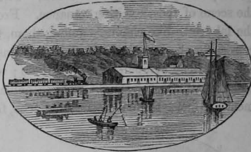
CAPE ST. VINCENT RAILROAD DEPOT.
