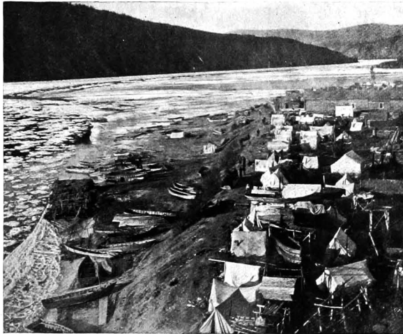
KLONDIKE "CITY"—KLONDIKE RIVER ENTERS ON THE RIGHT
