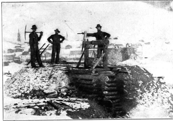
A DUMP, WITH A WINDLASS RAISED ON CRIB-WORK
