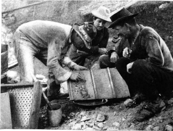
MAKING A "CLEAN-UP" FROM A ROCKER
