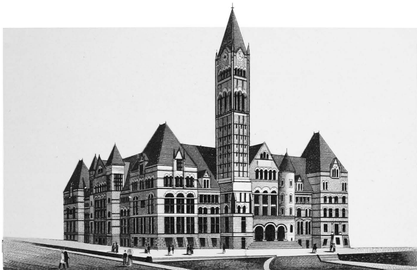
NEW MUNICIPAL AND COUNTY BUILDINGS.
