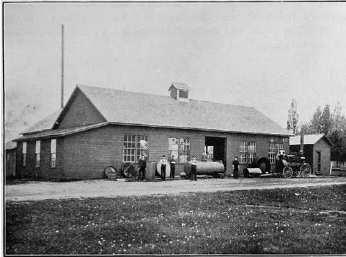
GODERICH STEAM BOILER WORKS, A.S.CHRystal, PROPRIETOR.
