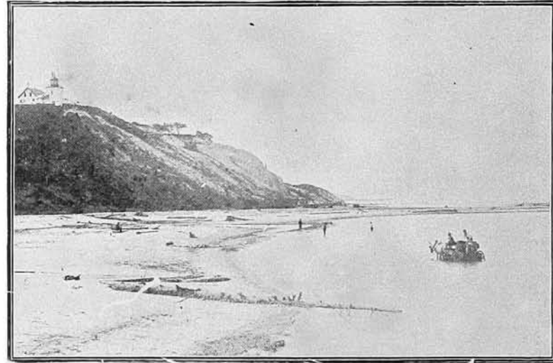
VIEW OF THE BEACH SOUTH OF THE HARBOR ENTRANCE
