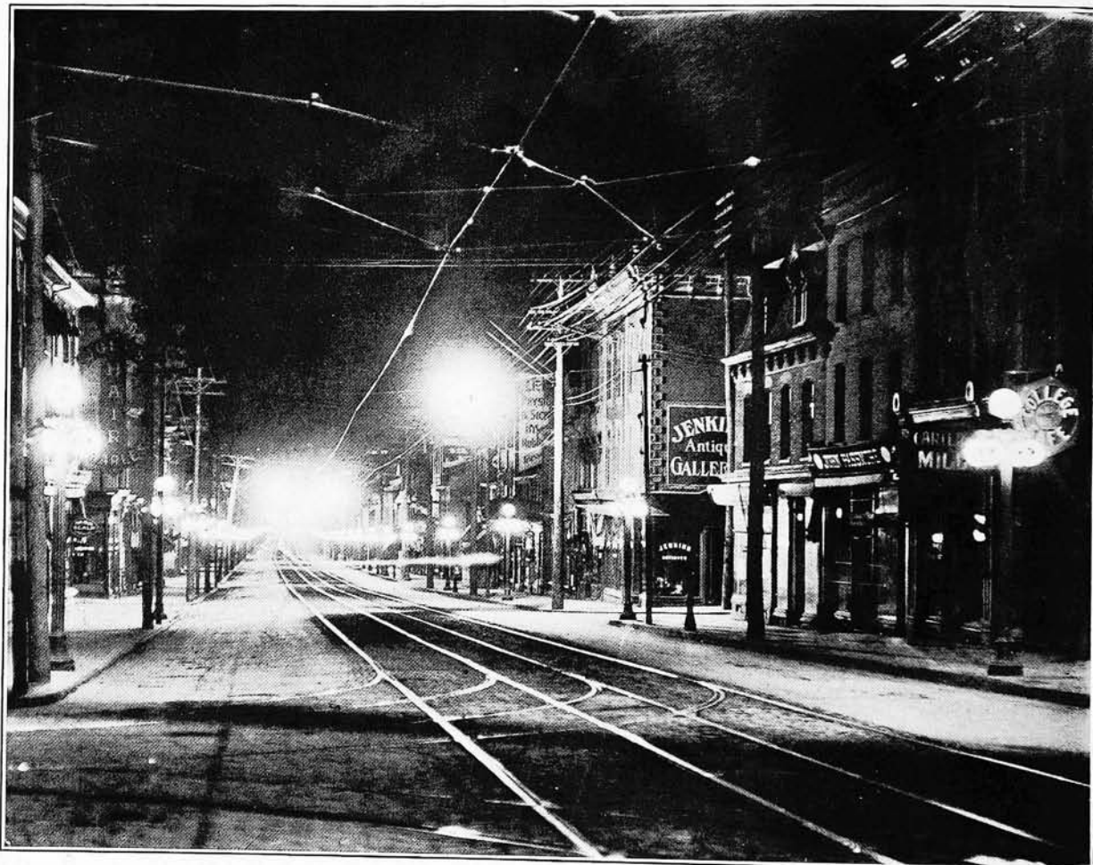
A Business Street showing the Cluster Lights of The Toronto Hydro-Electric System
