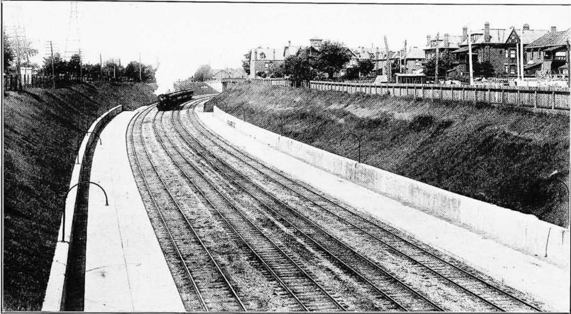
Grand Trunk Railway System's approach to the city of Toronto
