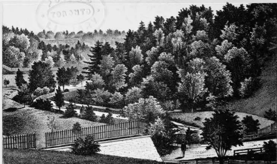
RESERVOIR NORTH TORONTO.
