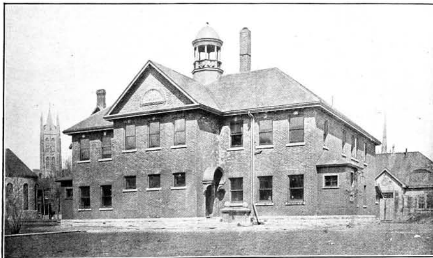
NEW DAIRY SCHOOL BUILDING.
