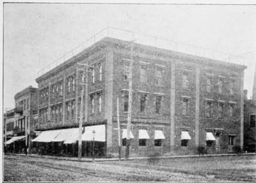
BANK OF COMMERCE, LAUTENSCHLAGER'S BLOCK,
