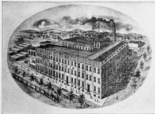
D. HIBNER & COMPANY'S FURNITURE FACTORY.
