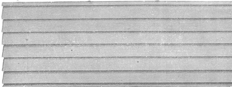
Fig. 39—Weatherboard Siding
