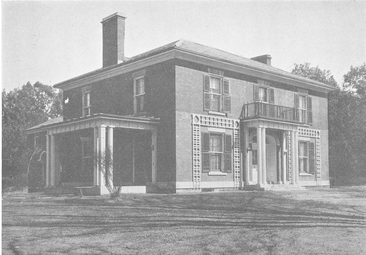
TRANSFORMATION OF AN OLD HOUSE IN BELLEVILLE By W. Breden Galbraith - Architect - Toronto
