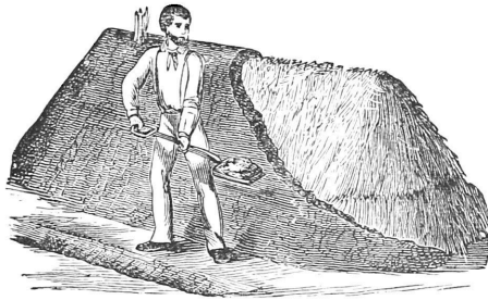
Fig. 243.—COVERING HEAP WITH EARTH.
