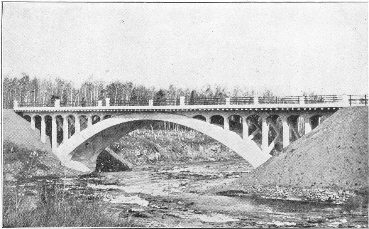
Concrete Bridge over Little Current River, Port Arthur, Ont.
