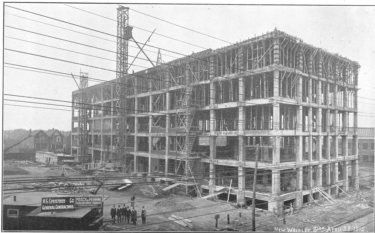
New Wrigley Building, Toronto, under construction
