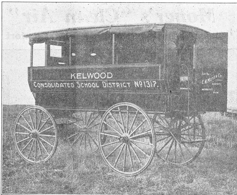
Exterior View With Curtains Rolled Up
