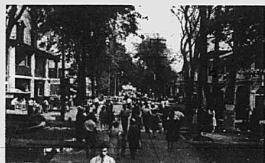
BUSINESS SECTION, CENTRE ISLAND, TORONTO, CANADA.
