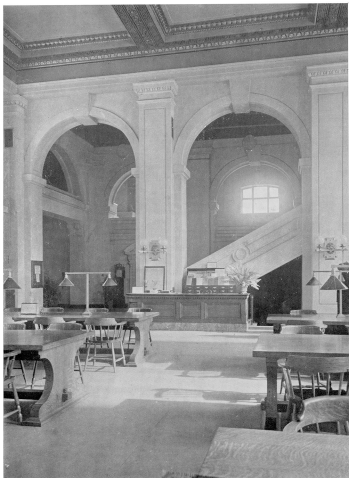
Interior of Reference Library, College Street, Toronto—Looking East
