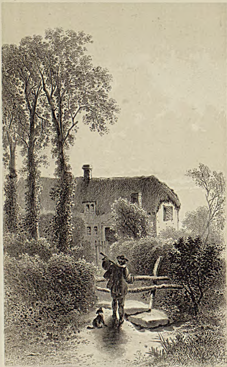
THE DAIRYMAN'S COTTAGE. NEAR ARRETON.
