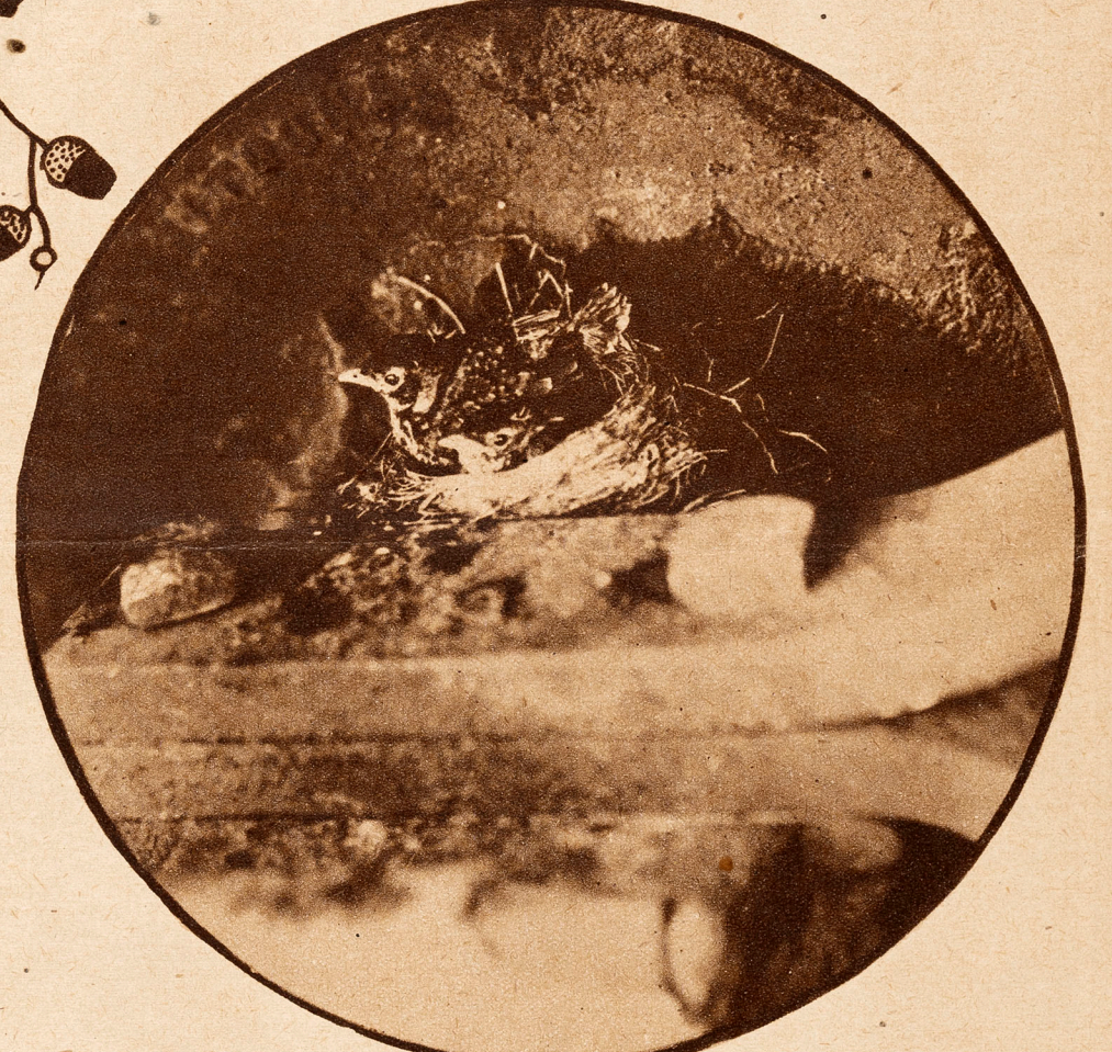
The journal-box of a freight car wheel was the odd place chosen by a robin for its nest. Just how the mother kept track of its young is a problem, for this car had been frequently moved around.
