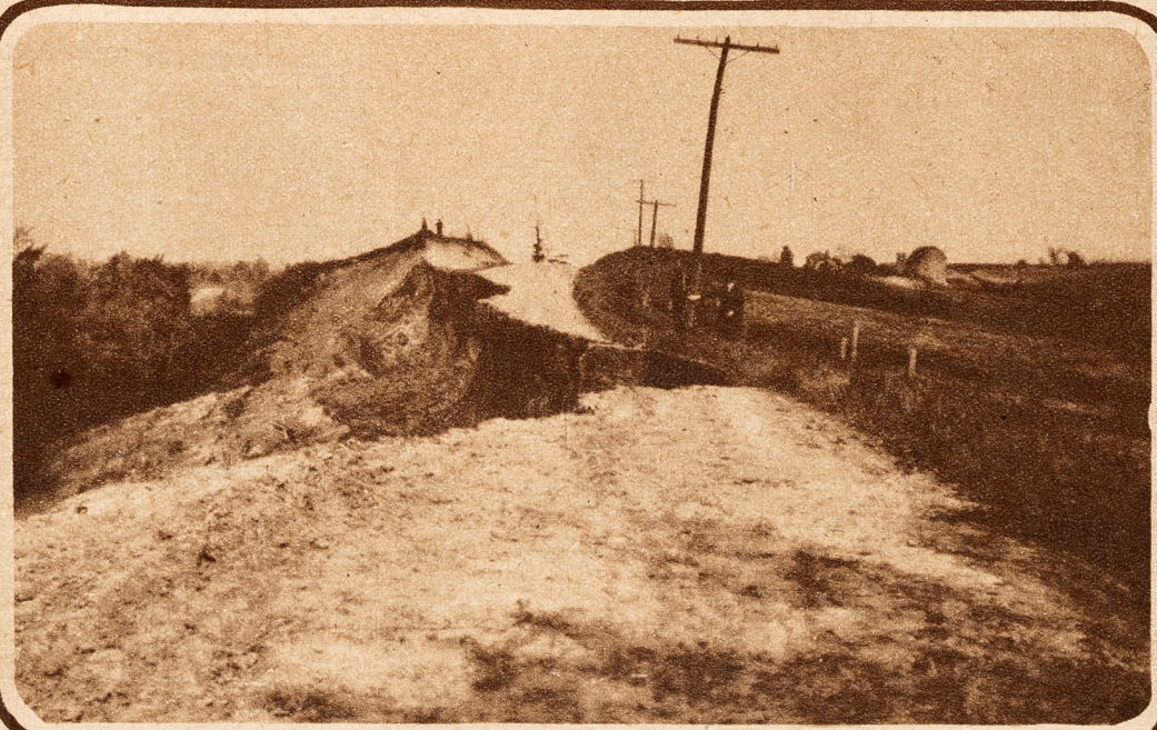
Landslide on river road between Brantford and Six Nations Indian Reserve, showing road running along brow of bluff cut in two by settling of large area. The picture on the right shows the extent of the fall in a graphic manner.
